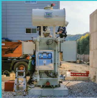
12.5 MVA, 22.9/10.5 KV, 60 Hz Power Transformer supplied to South Korea.
