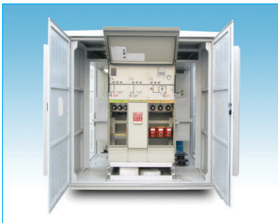
VIEW OF USS FROM HT COMPARTMENT SIDE
