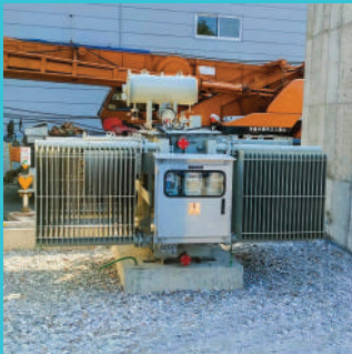
1.6 MVA, 10.5/0.46 KV, 60 Hz. Auxiliary Transformer Supplied to South Korea
