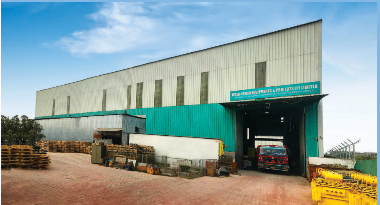
Manufacturing Unit 2 Tesla Power Equipments & Projects (P) Ltd. (Distribution Transformer Division)
