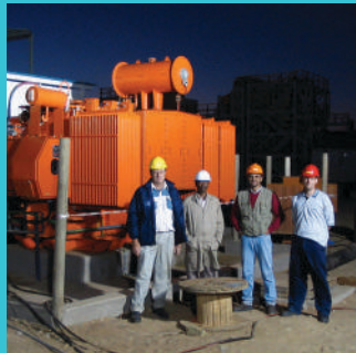
7.5 MVA, 33 KV Transformer installed at De Beers Diamond Mine, Namibia
