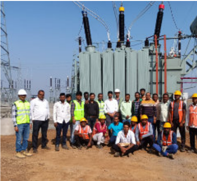
50 MVA, 220-33 KV Power Transformer
