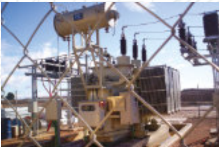
10-12.5 MVA 66-20KV UTE SOLAR-SS to Spain.
