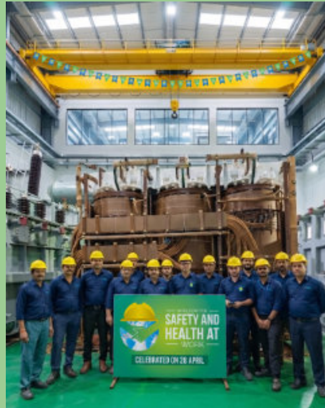
50 MVA-132kV CC Assembly
