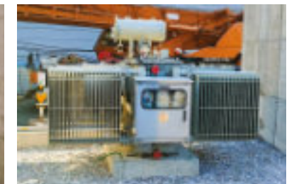
12.5 MVA, 22.9/10.5 KV, 60 Hz Power Transformer supplied to South Korea.
