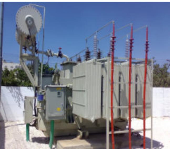
2 MVA 27.6 x 0.6KV Supplied to Canada
