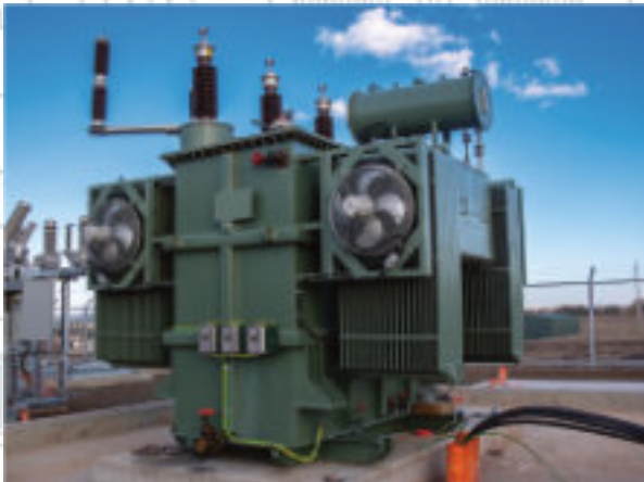
12.5 MVA 66 kV supplied to Australia
